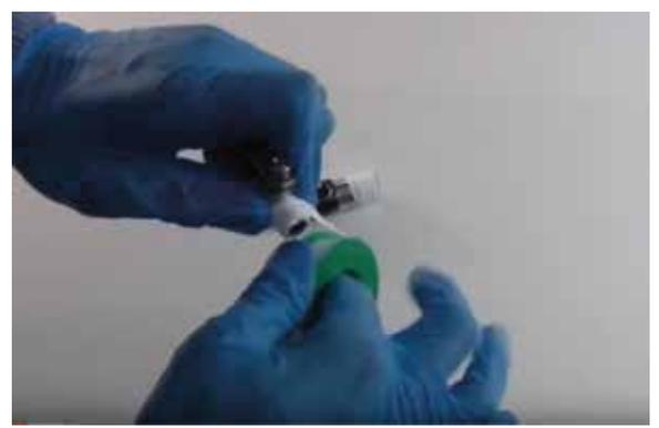
3) Then using your spanner, screw the ball valve into the feed in valve and tighten it with your spanner.
