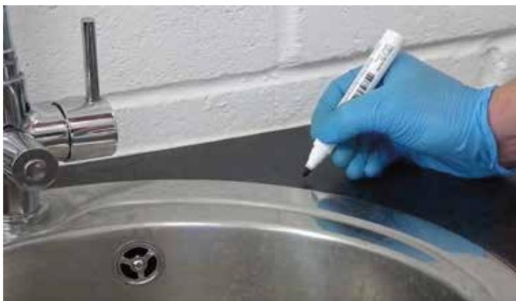
Ensure a flat surface available under on the other side of the worktop before marking the place the drill the hole for the tap. This is to ensure that the tap fixings which tighten the tap underneath have a clean flat surface to screw up against.
