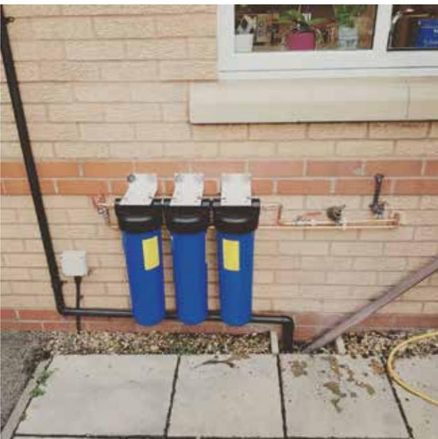
FIG 3: An example external installation before weatherproofing
