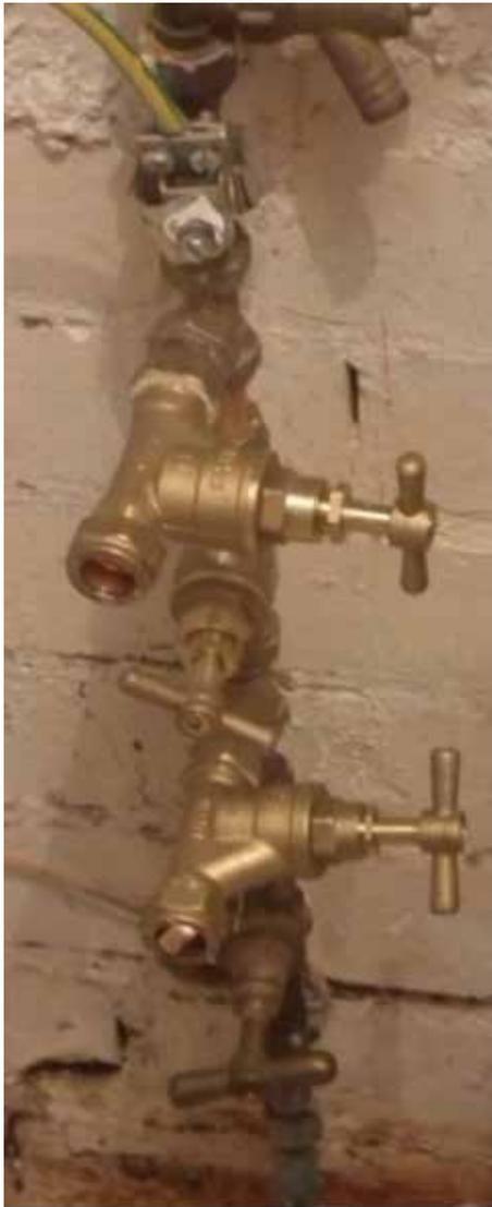
The next step is to make your bypass assembly and do all the necessary pipework to run pipes to the inlet and outlet of your system.
