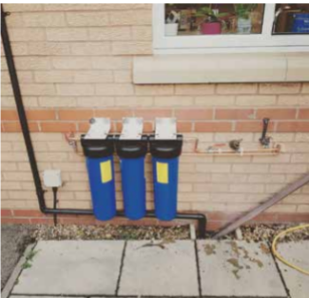
FIG 3: An example external installation before weatherproofing
